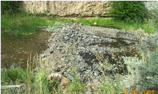
Using heavy equipment (right), irrigators push up streambed gravels to create tributary (right), cross-channel, (middle), and side-channel “push-up” dams for the purpose of creating deep pools for irrigation withdrawals in the Lower North Fork John Day River. (Photographs: Courtesy of the North Fork John Day Watershed Council and the Monument Soil and Water Conservation District)
