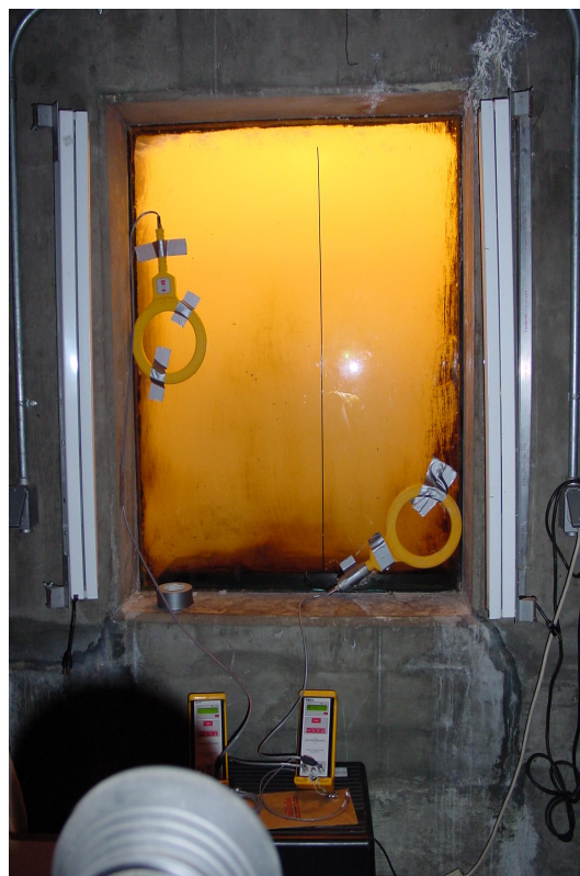
Migration timing of salmonid smolts is monitored via by this PIT Tag detection system at the Three Mile Falls Dam East. (Photograph: Courtesy of the Oregon Department of Fish and Wildlife)
