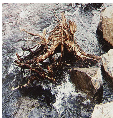
To improve pool quality and quantity, the Columbia Soil and Water Conservation District has installed rootwad revetment (left), large organic debris placement (middle), and vortex weirs (right), in the Tucannon River. (Photographs: Courtesy of the Columbia Conservation Soil and Water Conservation District)
