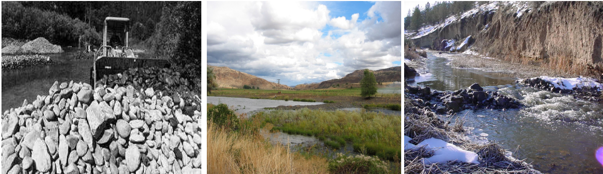
Using heavy equipment (right), irrigators push up streambed gravels to create tributary (right), cross-channel, (middle), and side-channel “push-up” dams for the purpose of creating deep pools for irrigation withdrawals in the Lower North Fork John Day River. (Photographs: Courtesy of the North Fork John Day Watershed Council and the Monument Soil and Water Conservation District)
