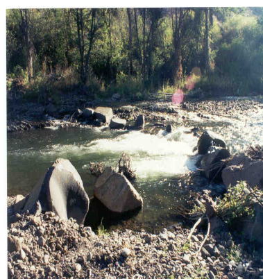
To improve pool quality and quantity, the Columbia Soil and Water Conservation District has installed rootwad revetment (left), large organic debris placement (middle), and vortex weirs (right), in the Tucannon River. (Photographs: Courtesy of the Columbia Conservation Soil and Water Conservation District)
