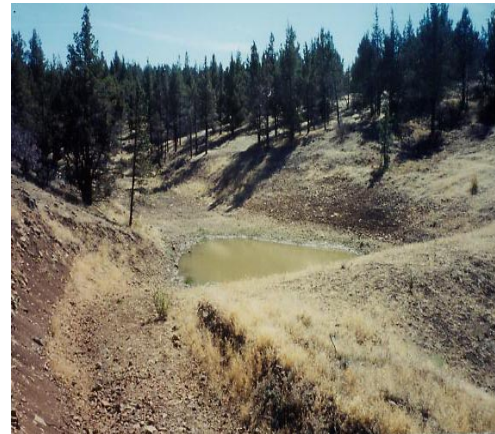
To reduce sediment (left) from entering tributaries in the Pine Hollow watershed, sediment control basins (right) have been created in the uplands. (Photographs: Courtesy of the Sherman County Soil and Water Conservation District)
