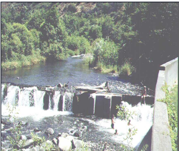
Prior to 1997, the Marie Dorian Dam (left) was a barrier to fish passage; however, in 1997 the Confederated Tribes of the Umatilla Indian Reservation removed the dam and restored fish passage (right). (Photographs: Courtesy of the Confederated Tribes of the Umatilla Indian Reservation)
