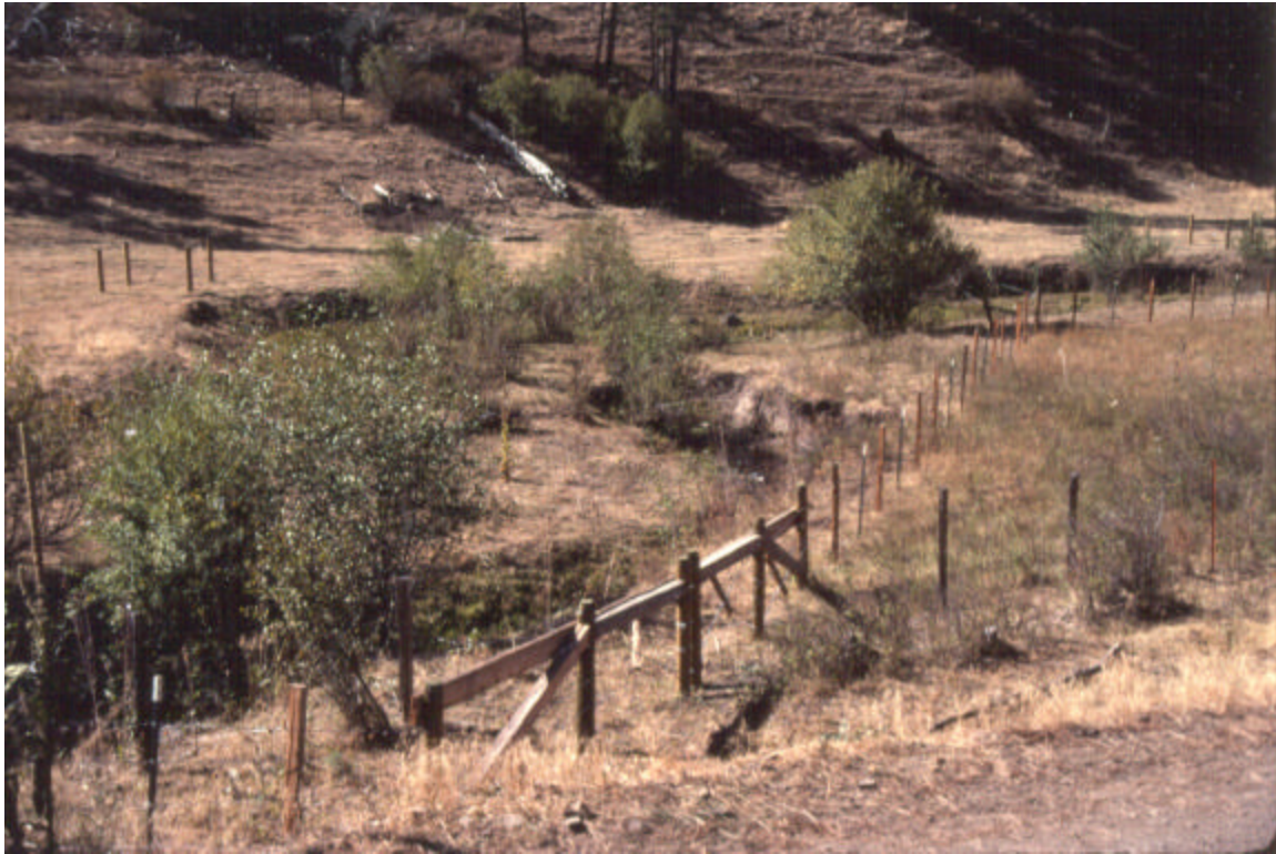
Butte Creek, McDaniel property, Photopoint #5, September 25, 1991. Vertical cut banks and only moderate amounts of riparian vegetation are evident. The newly constructed fence on the right bank appears to have been placed too close to the streambank.
